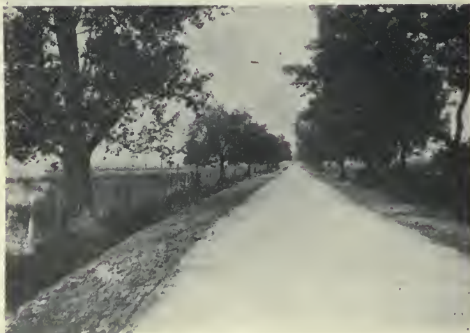
Banlieue to Three Rivers—Concrete laid in 1915.
